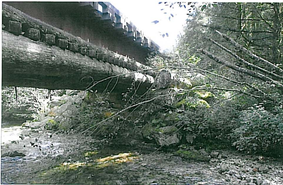
CK-2270 Right abutment
